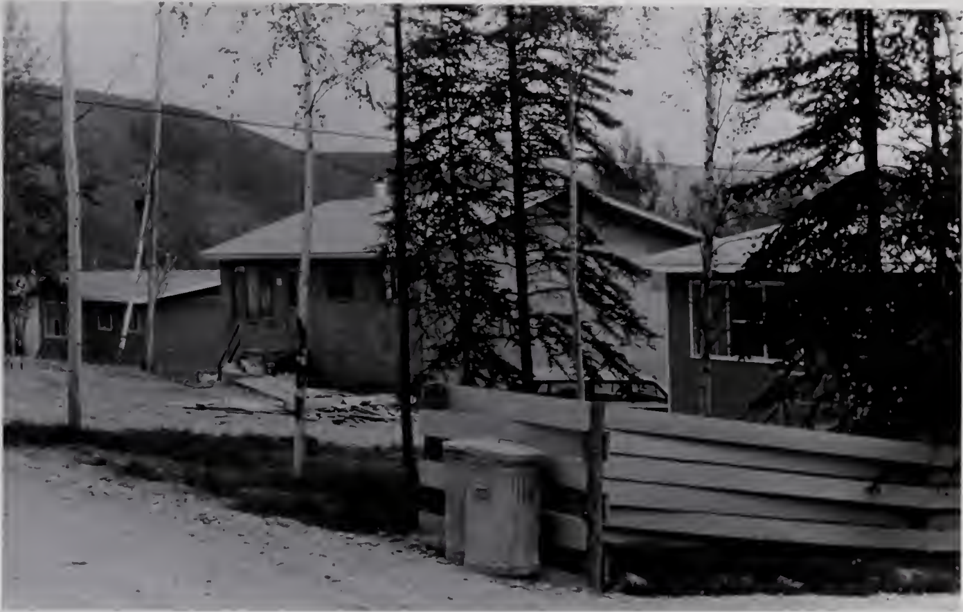
Plate 7. Typical housing in Clinton Creek. The houses to the right and left are prefabricated. The unfinished house in the center has been roughed in by the company and is being completed by the employee-owner. (July 1970).
